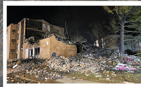
Lyttonville Road Explosion
