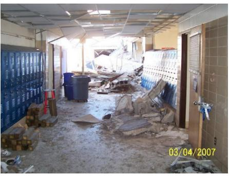
Photo from inside Enterprise High School in Alabama after the March 1, 2007, tornado. This is where many of the eight children were killed when the walls and roof collapsed. Photo Credit: Dothan-Houston County (AL) EMA
