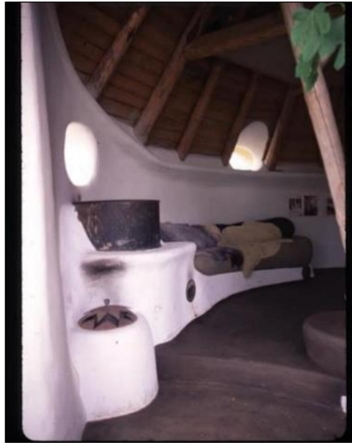
Serving as a Thermal Battery the cob bench can store heat for several days, radiating it out slowly,
